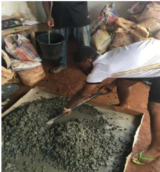
Plate 3.2 Hand mixing of the concrete
