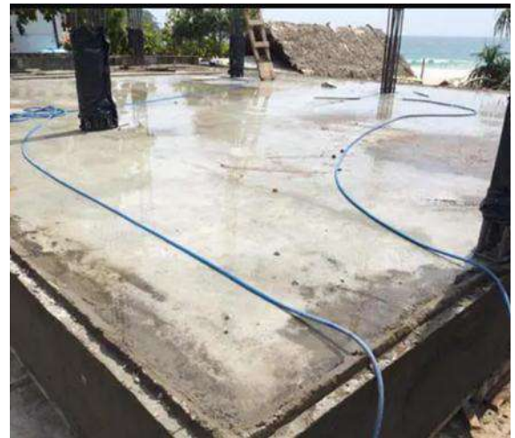
Fig 2.5b Curing by ponding
