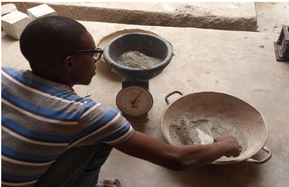
Plate 3.14: Batching of cement with the use of a measuring scale
