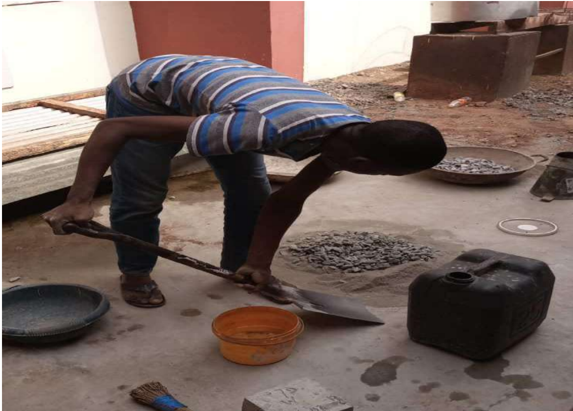
Plate 3.15: Mixing of concrete constituents together
