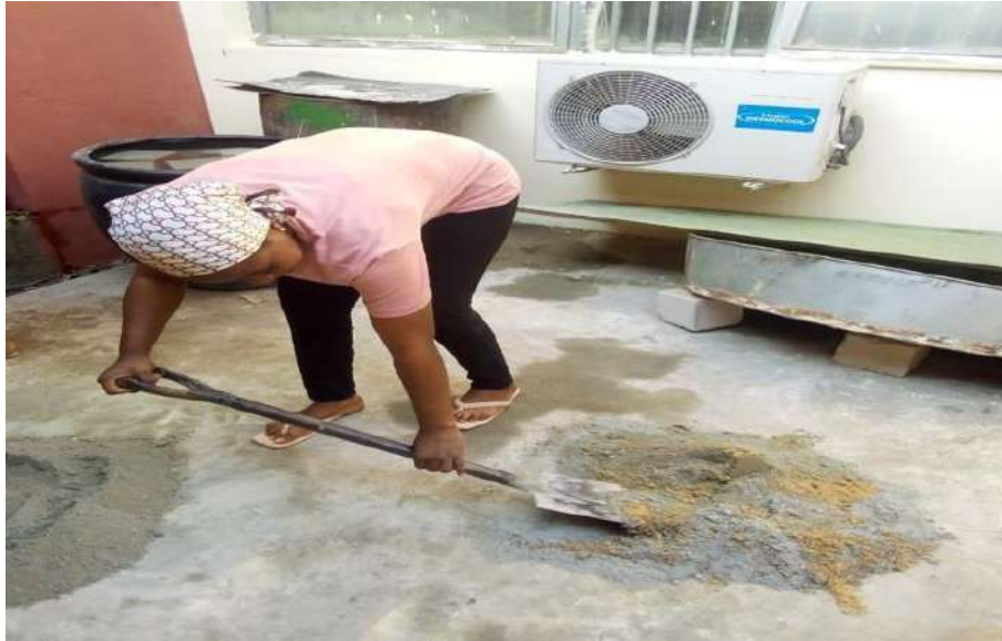
Plate 3.3: Hand mixing of concrete
