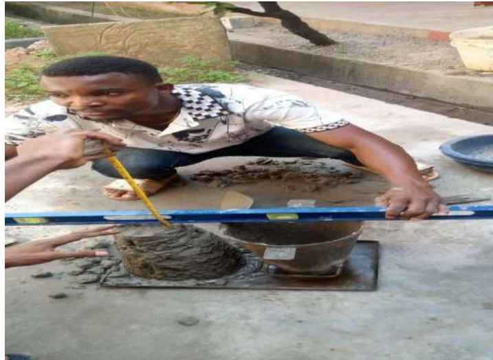
Plate 3.4: Slump test in progress
