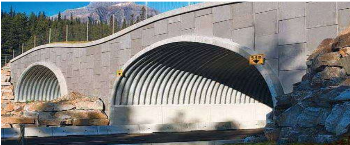
Plate 2.8.1 Steel Arch Culvert (Source: http://www.visitgrey.ca ).
