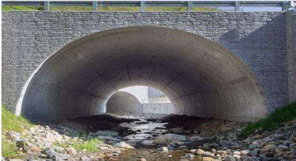
Plate 2.6 Single Concrete Pipe Arch Culverts (Source: http://www.visitgrey.ca ).
