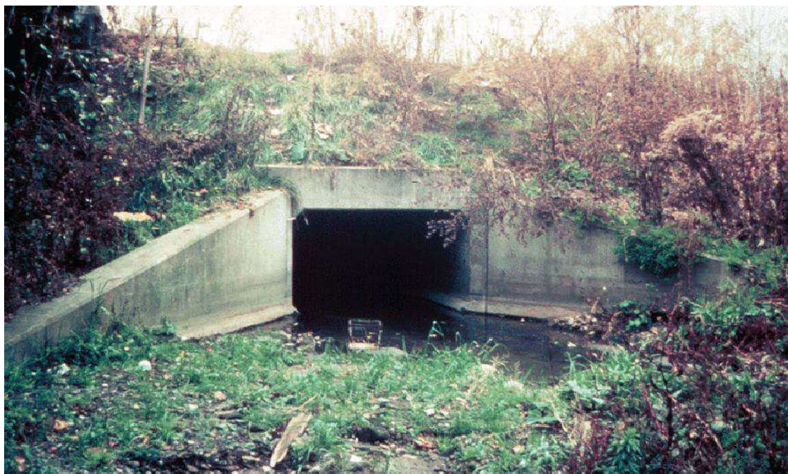
Plate 2.3 Single Concrete Box Culvert (Source: miller-miller-inc.com).
