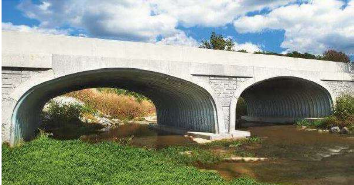
Plate 2.8 Reinforced Concrete (RCC) Arch Culvert (Source: http://www.visitgrey.ca ).
