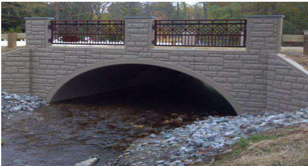
Plate 2.7 Single Concrete Pipe Arch Culvert with a small Channel (Source: http://www.visitgrey.ca ).
