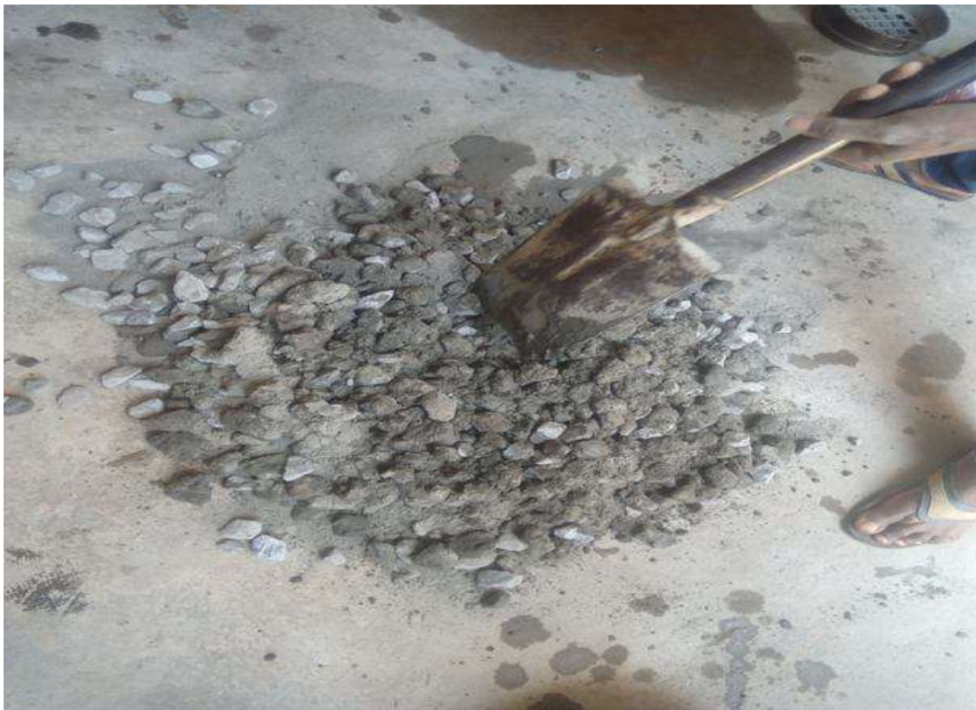
Figure 3.6: Mixing of concrete
