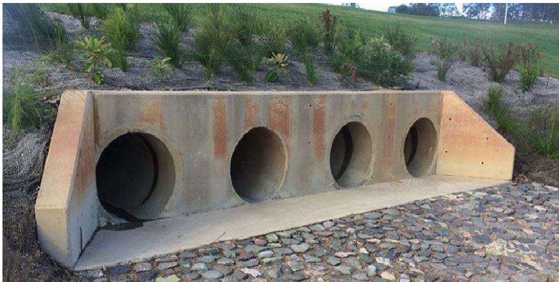
Plate 2.0 Multiple Pipe Culvert (Source: metal-culvert.com).
