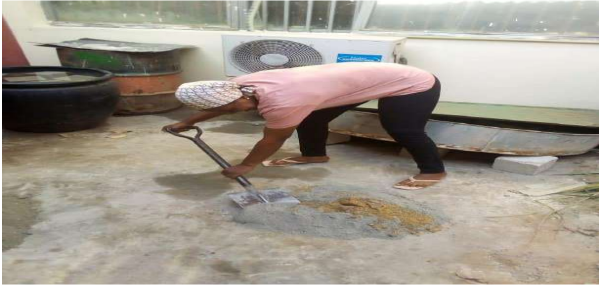
Plate 3: Batching of Concrete.
