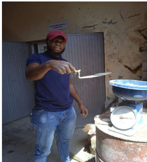
Plate 3.7: Batching of concrete
