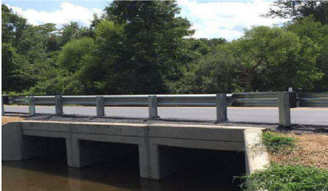
Plate 2.5 RCC Solid Slap Culverts. (Source: http://www.visitgrey.ca ).
