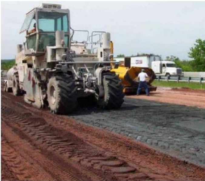
Plate 1: A road reclaimer mixes soil with moist conditioned fly ash (Beeghly, 2003).
