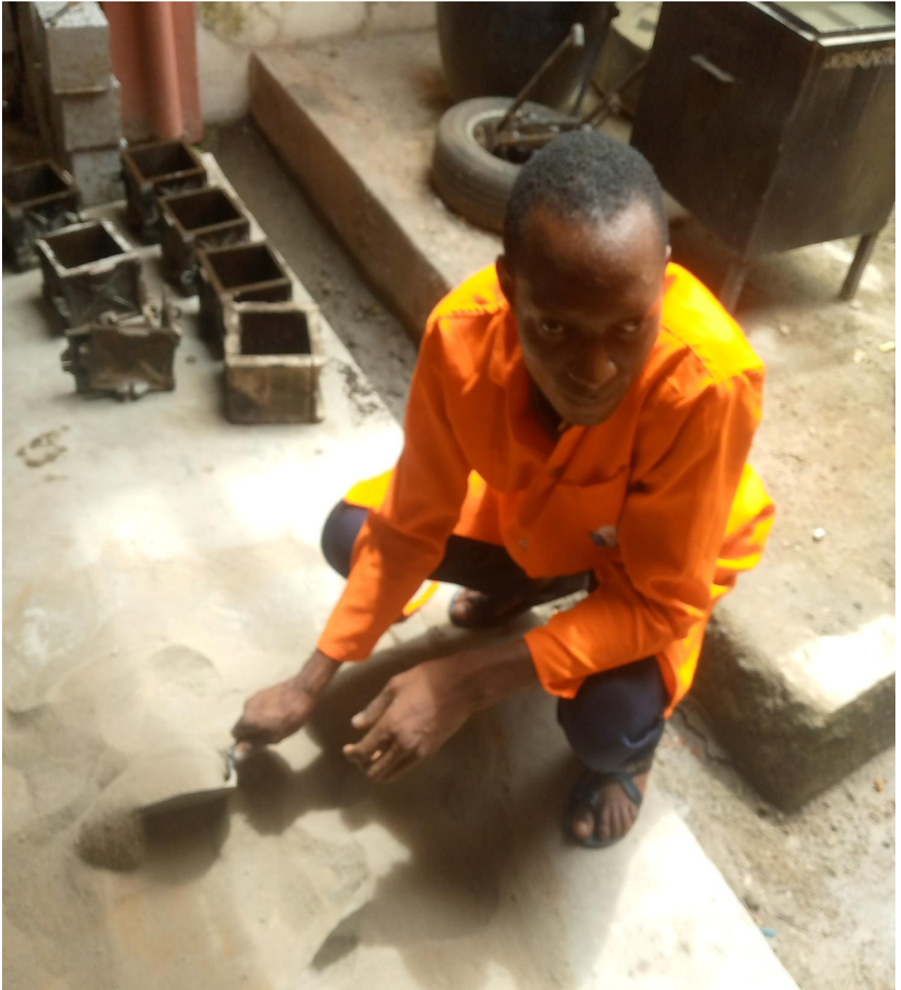
Fig 3.1: Mixing materials and block moulding.
