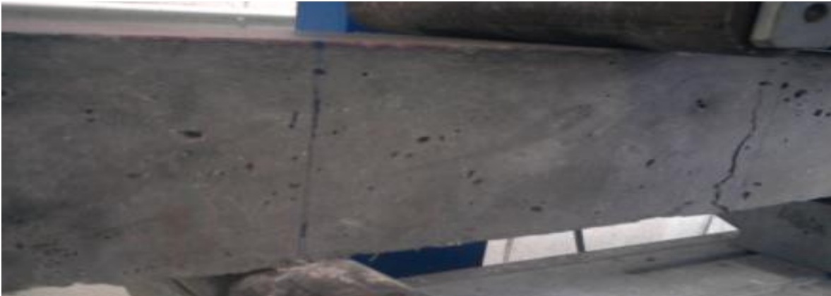
Figure 4.14: Failure Mode of Pop Fiber Reinforced Concrete
