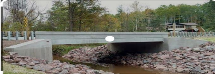
Fig. 5 RCC Solid Slab culvert (Daily Civil, 2023).
