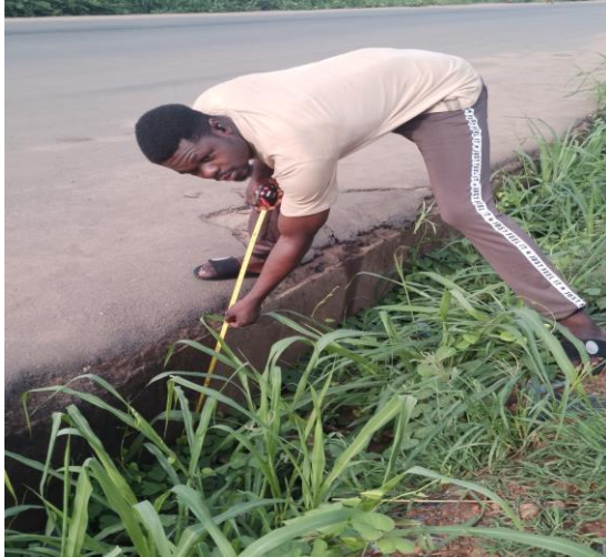
Plate 1: Field measurements of the dimensions of the Culvert along Enugu-Onitsha Expressway.
