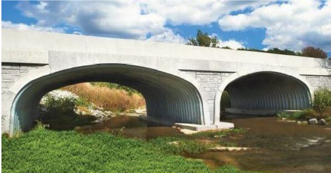
Plate 2.8 Reinforced Concrete (RCC) Arch Culvert (Source: http://www.visitgrey.ca ).
