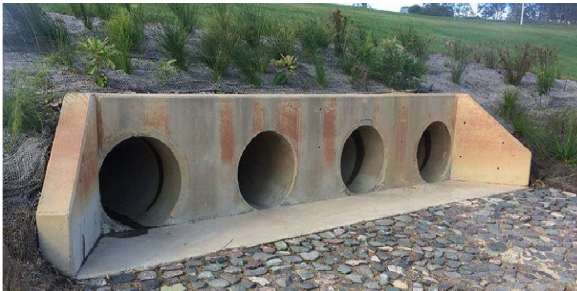
Plate 2.0 Multiple Pipe Culvert (Source: metal-culvert.com).
