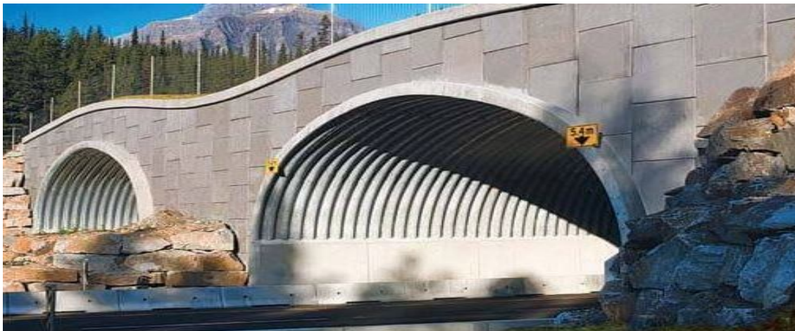
Plate 2.8.1 Steel Arch Culvert (Source: http://www.visitgrey.ca ).
