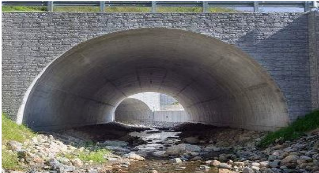
Plate 2.6 Single Concrete Pipe Arch Culverts (Source: http://www.visitgrey.ca ).
