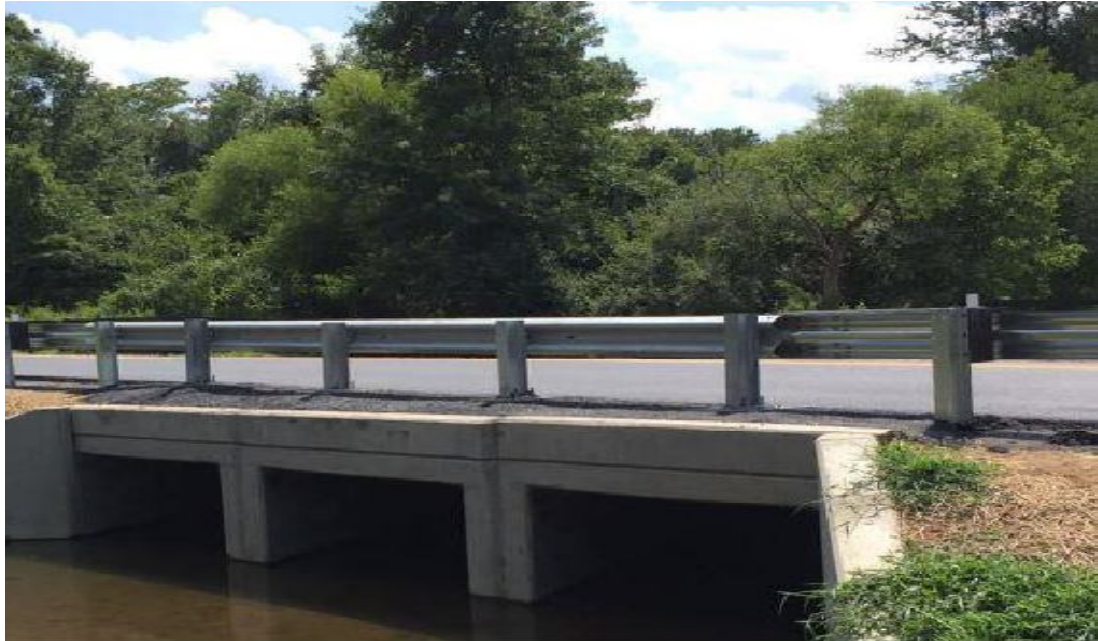
Plate 2.5 RCC Solid Slap Culverts. (Source: http://www.visitgrey.ca ).
