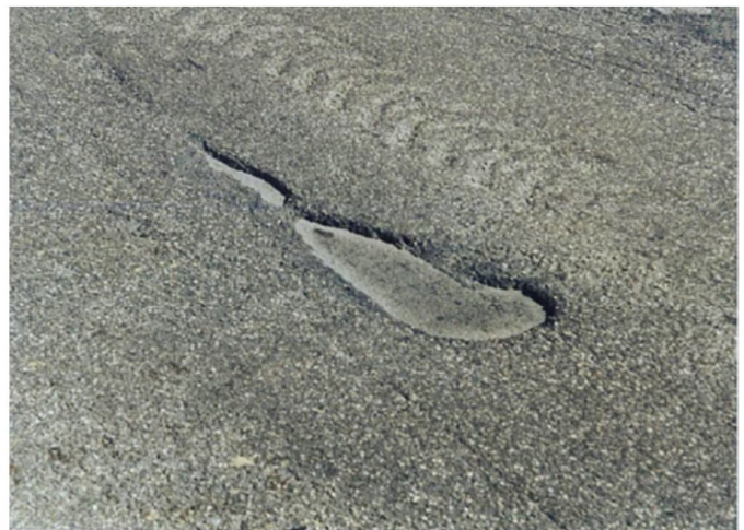
Fig. 8: Medium Severity of Debonding Distress in Flexible Pavement [12]
