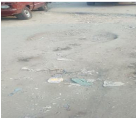
Fig.12: High Severity of Raveling distress on Forestry flexible road pavement
