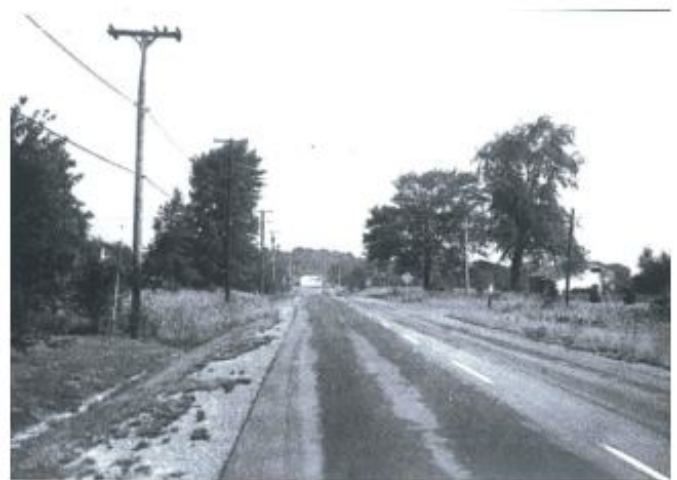
Fig. 5: High and Medium Severity of Bleeding Distress in Flexible Pavement [12]
