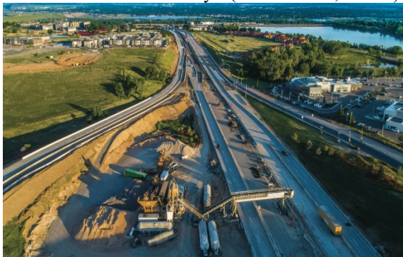
Plate 3. Crushing Plant Used to Produce RCA for Concrete Pavement (Source: Cavalline et al., 2022)
