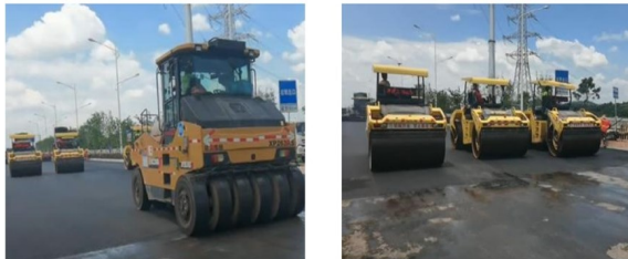
Plate 2. Schematic Diagram of Unmanned Rolling (Source: Yuan et al., 2012).
